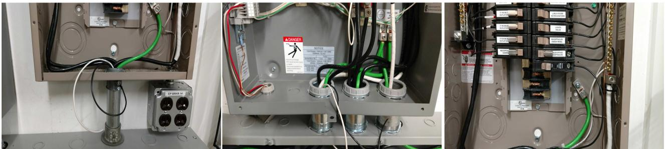
3. Using 5 self tapping screws, install the M328V2. Connect the load side power to the load side connection on the board. For this example we are connecting line to neutral. Polarity is labeled on the power supply. For a line to line installation polarity does not apply.
