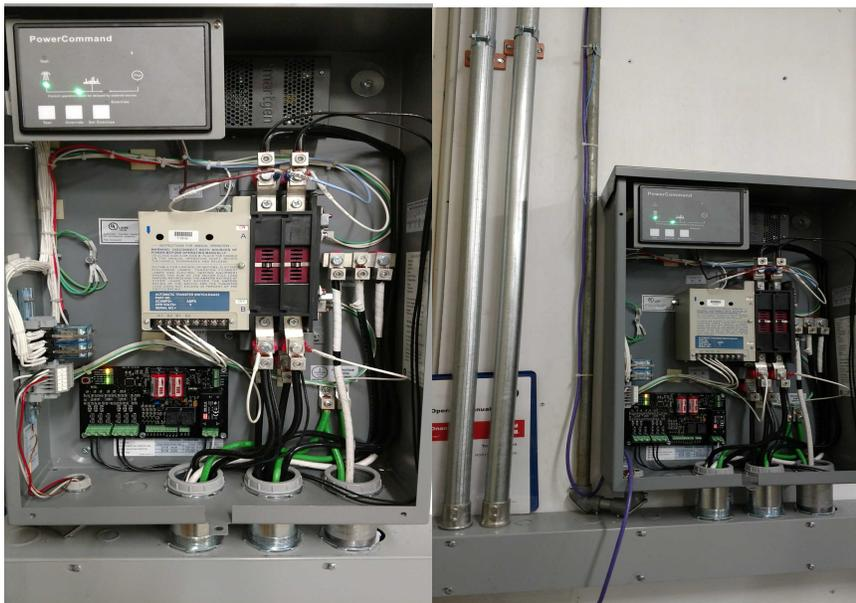
5. Now that all of the high voltage connections are complete, run a low voltage connection for the modem and route the wire thru the transfer switch. For the modbus connection, belden shielded twisted pair is recommended. In this installation we are using standard CAT 5E ethernet cable.
