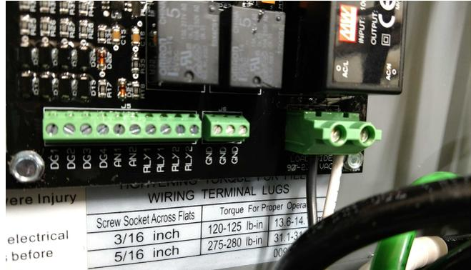
4. Install connections for single phase line to line on both generator and utility using terminals A and B. Route these connections to the corresponding lugs on the transfer switch.
