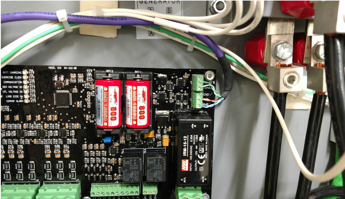
9. Check all wiring before plugging in the modem. If you are using the ethernet module, plug in the ethernet connection before applying power to the modem. Plug in the main power connector .
