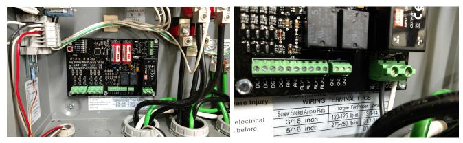
4. Install connections for single phase line to line on both generator and utility using terminals A and B. Route these connections to the corresponding lugs on the transfer switch.
