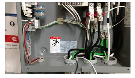
2. For convenience, install a breaker in the load side panel and run a power connection from the emergency panel to the transfer switch. This will make it easy to hard reset the M328V2 if needed.
