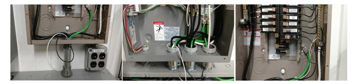
3. Using 5 self tapping screws, install the M328V2. Connect the load side power to the load side connection on the board. For this example we are connecting line to neutral. Polarity is labeled on the power supply. For a line to line installation polarity does not apply.
