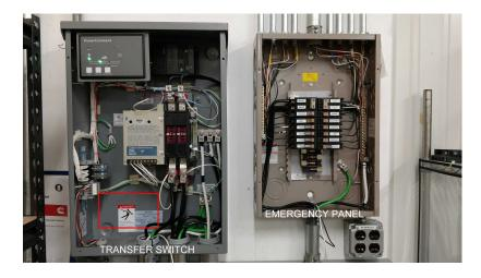
First locate a flat surface clear of any existing wiring. In this transfer switch the lower left corner is available with minimal modifications.
