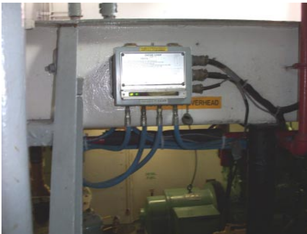
Details: Flight Systems' Model 550 Engine Saver ® installed to provide protection for the Lady Jill's starboard Volvo 400hp Diesel.
